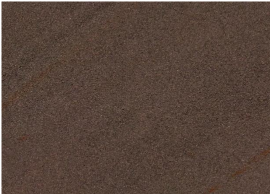
9) 57 – Weathering Low, Asphalt – Section T5
