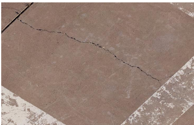
11) 63 – Longitudinal, Transverse, and Diagonal Cracking Medium, Asphalt – Section H1a
